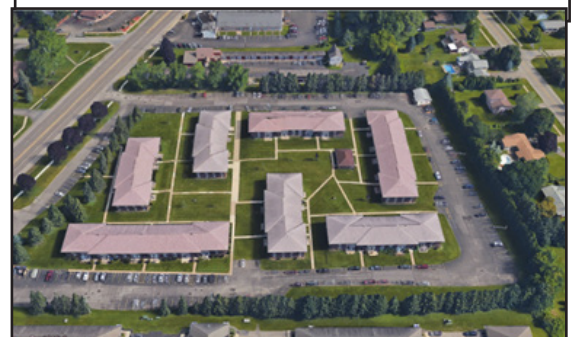
These aerial images demonstrate some of the residential development types and patterns found in Penfield.
